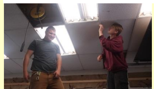
Installing new ceiling tiles
